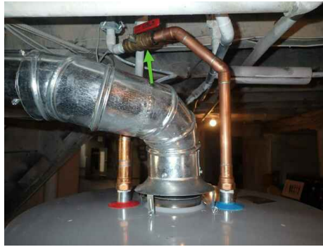
Water Shutoff Valve
