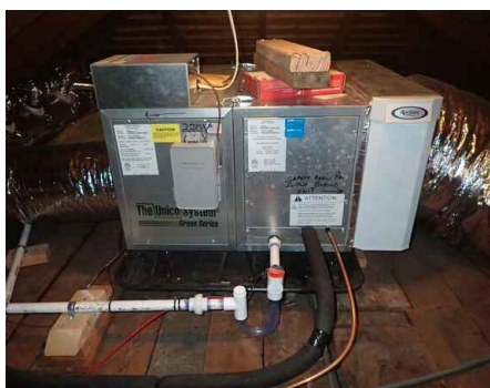
Air Handler/Evaporator Unit
