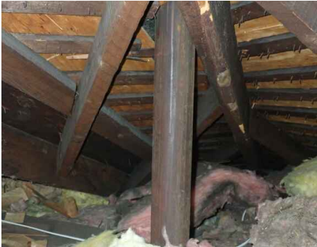
Plumbing Vent Stack
